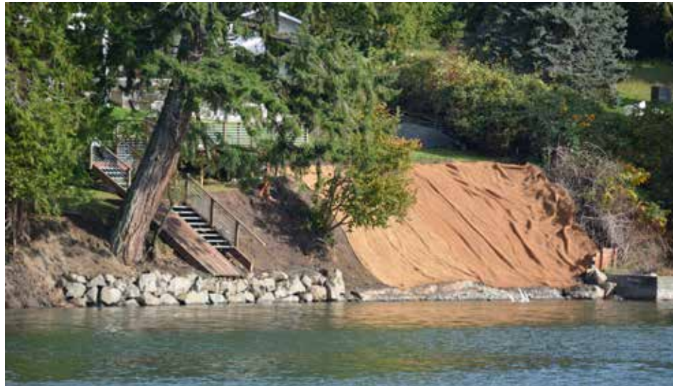
Soft shoreline after reconstruction
